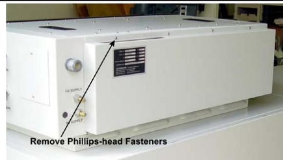
Figure 3-2 Lower rear access panel
