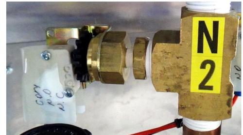
**Figure 2-53 IPS Inlet Pressure Switch**
