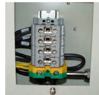
Figure 2-18 380-415Vac, 3PH 4-wire
