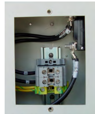
Figure 2-16 1-PH Connection
