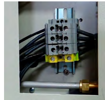
Figure 2-17 208-240Vac, 3-PH, 4 wire
