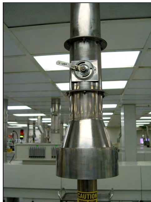
Figure 2-31 Exhaust Connection Detail
