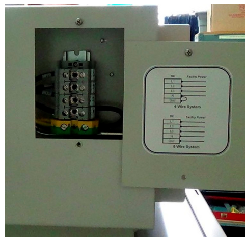
Figure 6-2 3-Phase Electrical (Option)
