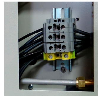
Figure 2-15 208-240Vac, 3-PH, 4 wire
