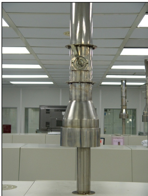
Figure 2-28 Exhaust Connection
