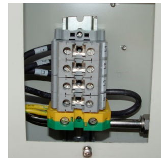
Figure 2-16 380-415Vac, 3PH 4-wire
