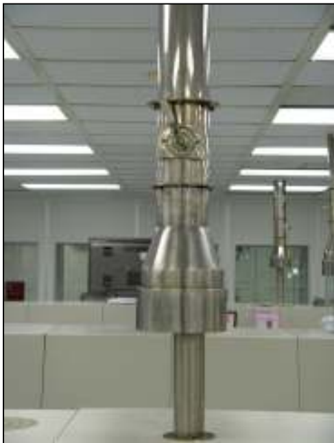
Figure 2-28 Exhaust Connection
