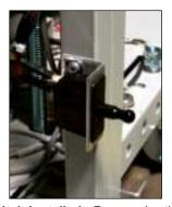
Panel Switch Installed - Bypass (out) Position
