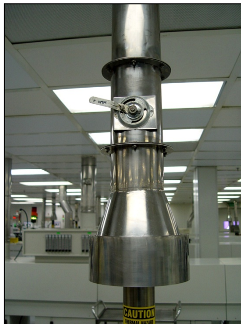
Figure 2-28 Exhaust Connection Detail
