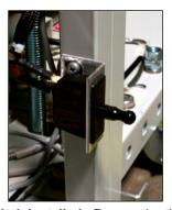
Panel Switch Installed - Bypass (out) Position
