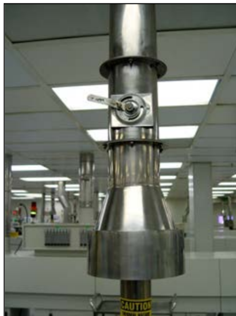
Figure 2-29 Exhaust Connection Detail
