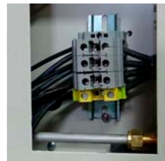
Figure 2-15 208-240Vac, 3-PH, 4 wire
