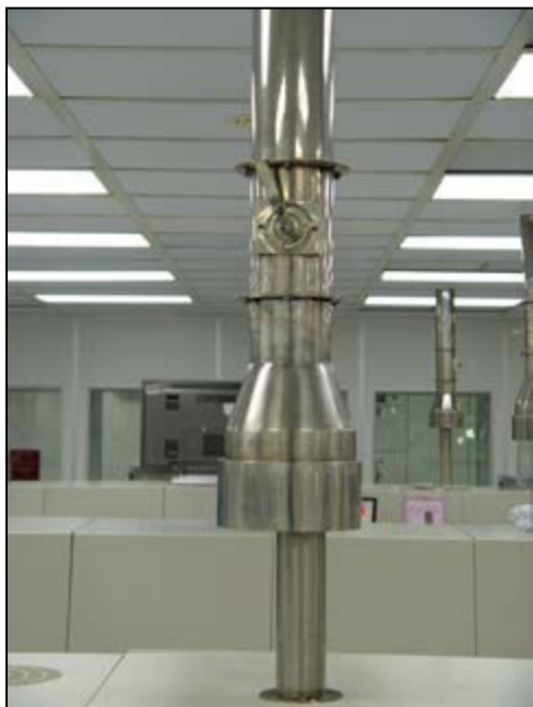
Figure 2-28 Exhaust Connection
