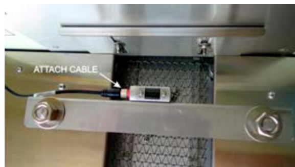
Figure 2-27 Connect SENSLAS cable
