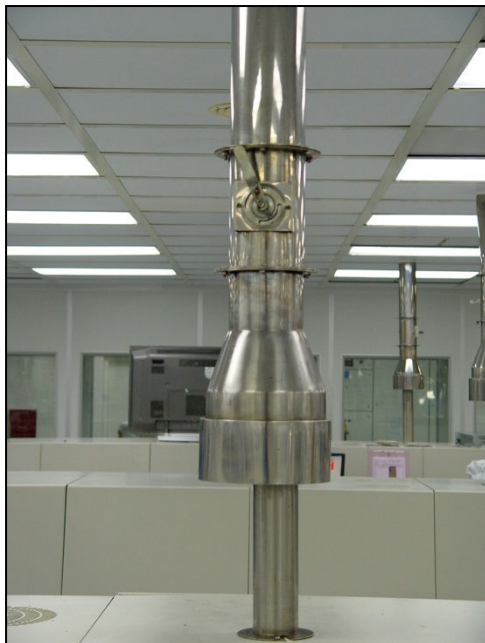
Figure 2-30 Exhaust Connection
