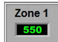
Figure 3-8 Zone Temperature display
