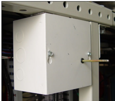
Figure 2-22 Interlock disconnect switch enclosure
