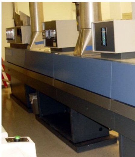
Figure 2-32 Cabinet Exhaust Example
