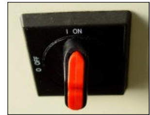
Figure 2-21 Interlock Disconnect switch
