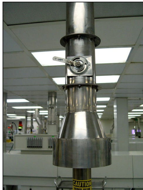
Figure 2-31 Exhaust Connection Detail
