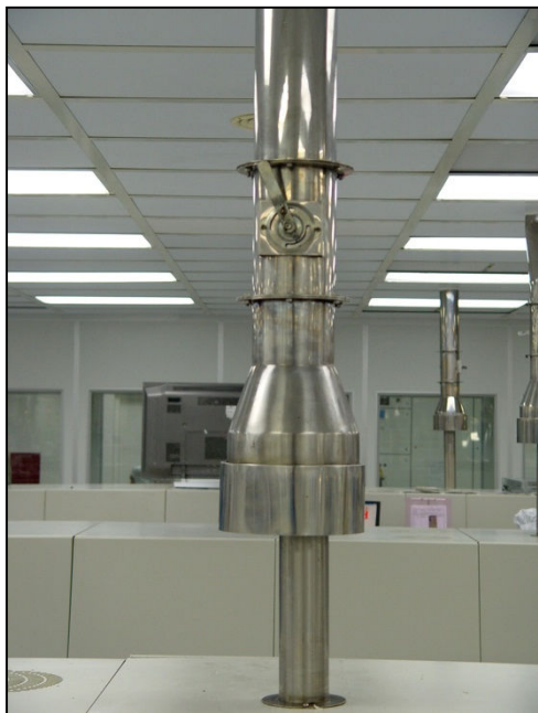
Figure 2-30 Exhaust Connection
