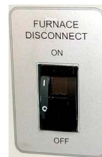
Figure 0-18 3-Phase Circuit Breaker
