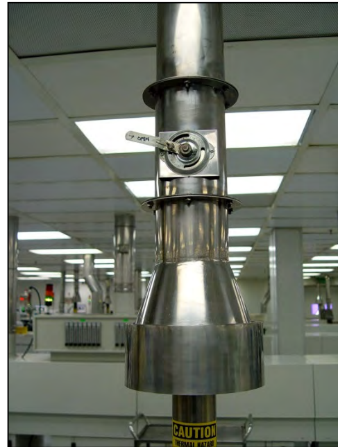
Figure 1.2.12 Exhaust Connection Detail
