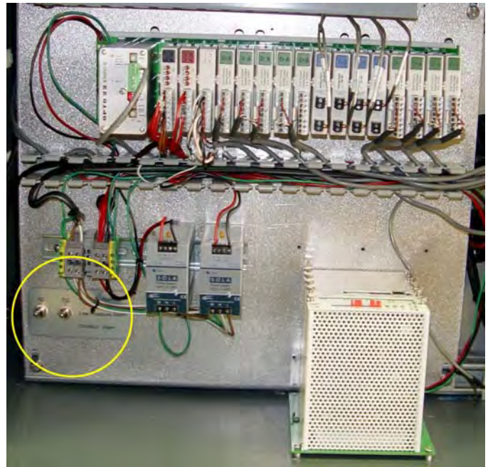
Figure 3.14.1 IPS Inlet Pressure Switch
