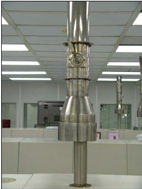
Figure 1.2.11 Exhaust Connection
