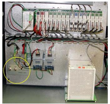
Figure 3.14.1 IPS Inlet Pressure Switch
