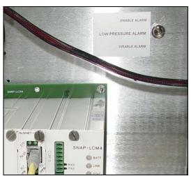
Figure 3.17.1 Enable Low Pressure Alarm switch
