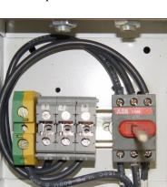
Figure 1.2.9 Disconnect Switch and Power Connection Terminal Blocks
