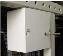
Figure 1.2.7 Disconnect Switch Enclosure
